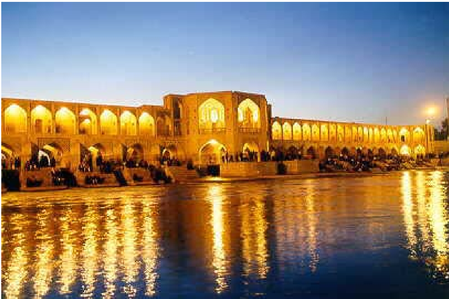
The Khaju bridge, the best known bridge in Esfahan
